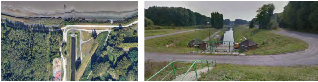
FIGURE 2-4 DISCHARGING STATION LOCATED N-E TO THE SITE
