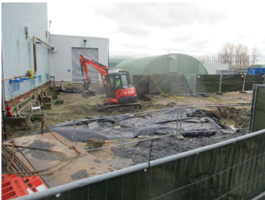
Backfilling and levelling
