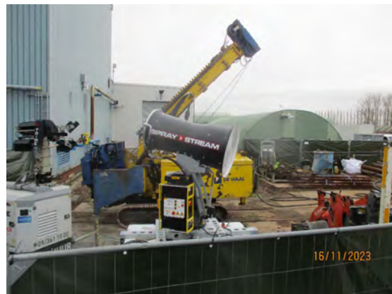
Mobilization and set-up drill rig
