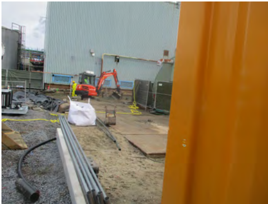
Backfilling and levelling
