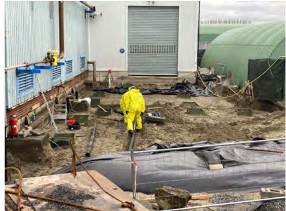
Installation of new sewer lines
