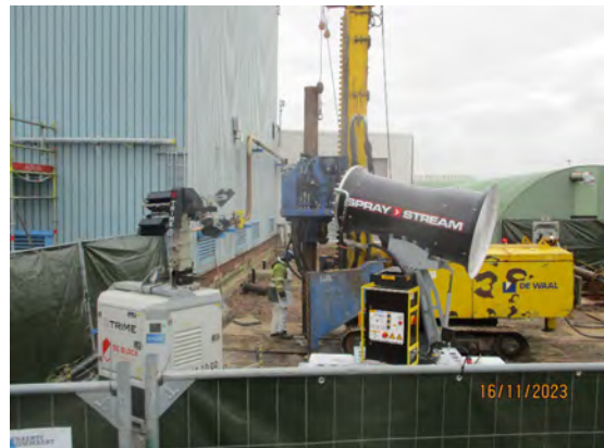
levelled and compacted work zone
