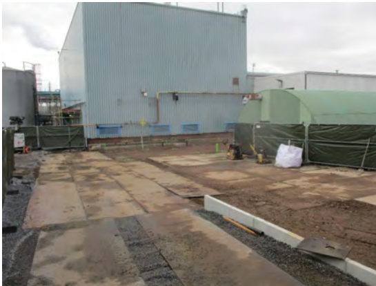
Work zone in the morning
