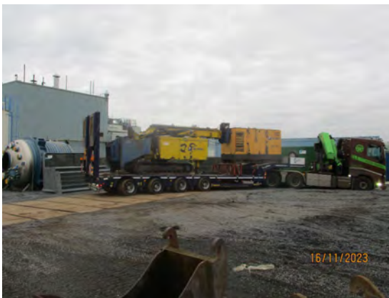
Mobilization and set-up drill rig
