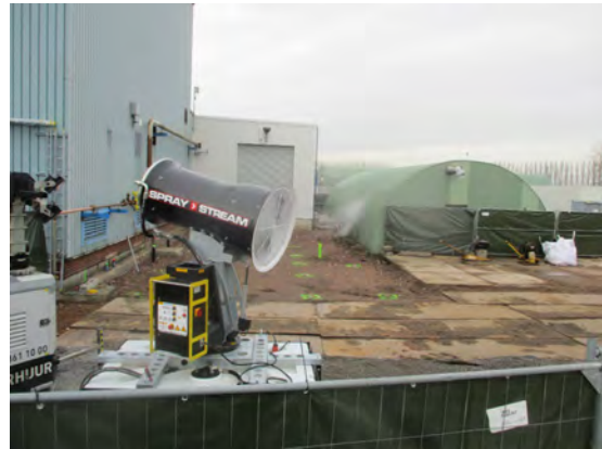
Work zone in the morning
