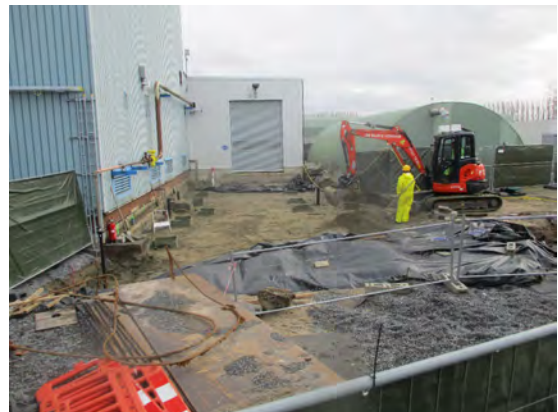
Backfilling and levelling
