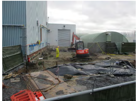
Backfilling and levelling
