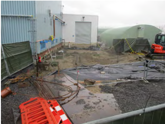
Installation of new sewer lines
